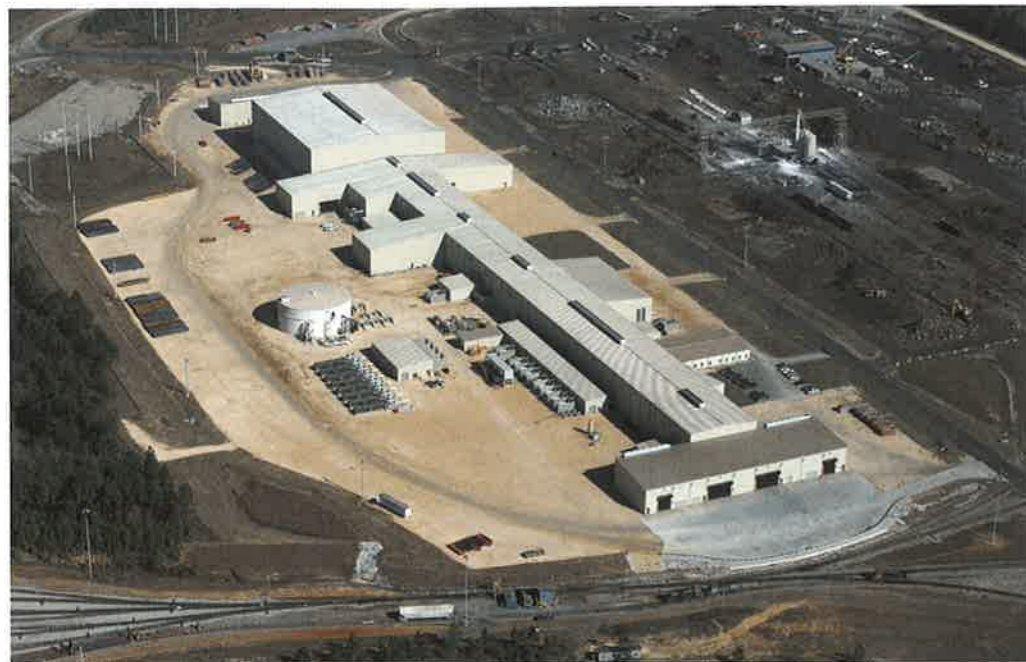
An expansion of the steelworks in Mobile, Alabama (USA) uses ten PROFINET controllers to control more than 650 field devices.
